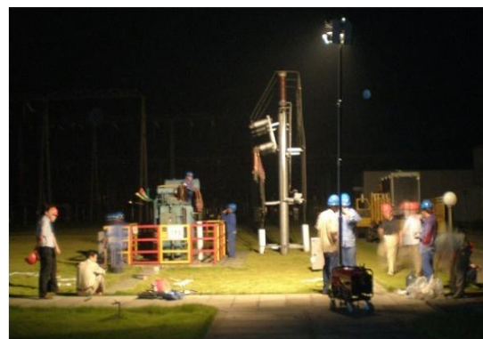
LED flood Light for city Center park project, 与FLS Lighting在中国
