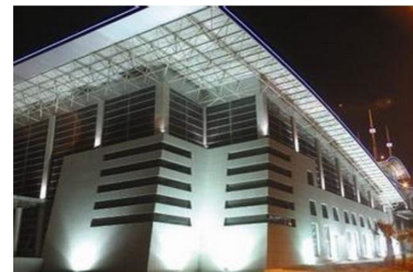
LED flood light, Museum lighting solution, 澳洲Gerard Lighting博物馆项目
